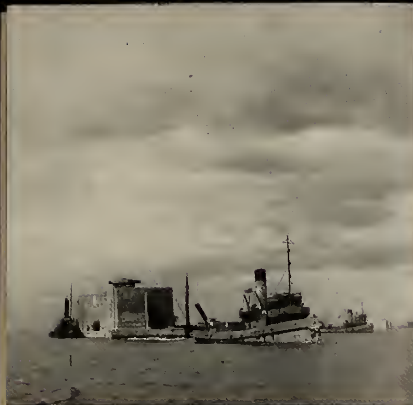
3. The parts were towed 100 miles across the stormy English Channel by tugs, protected by the Royal Navy. Here is seen one of the 150 concrete caissons which formed the main breakwaters, being towed.
